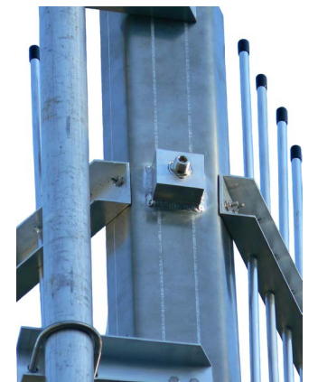
N-type female jack in rear of dipole assembly.
